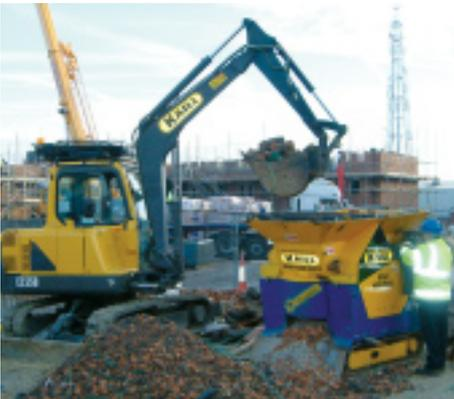
Crushing machine for brick and block waste, producing hardcore for use elsewhere on the Redrow development at Stamford Brook, Altrincham.
